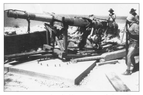
BEACON Battery, Garden Island in 1943. A US 4 inch 50 calibre Mk IX Model 5 or 6 Naval gun is manoeuvred onto its mounting. (Photo Major M A Primrose)
